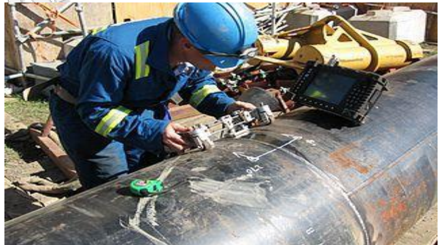
Ultrasonic Weld Inspection:
