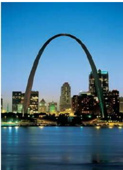
Glen Allison/Stone/Getty Images The design of the Gateway Arch near St. Louis is based on an inverted hyper-
