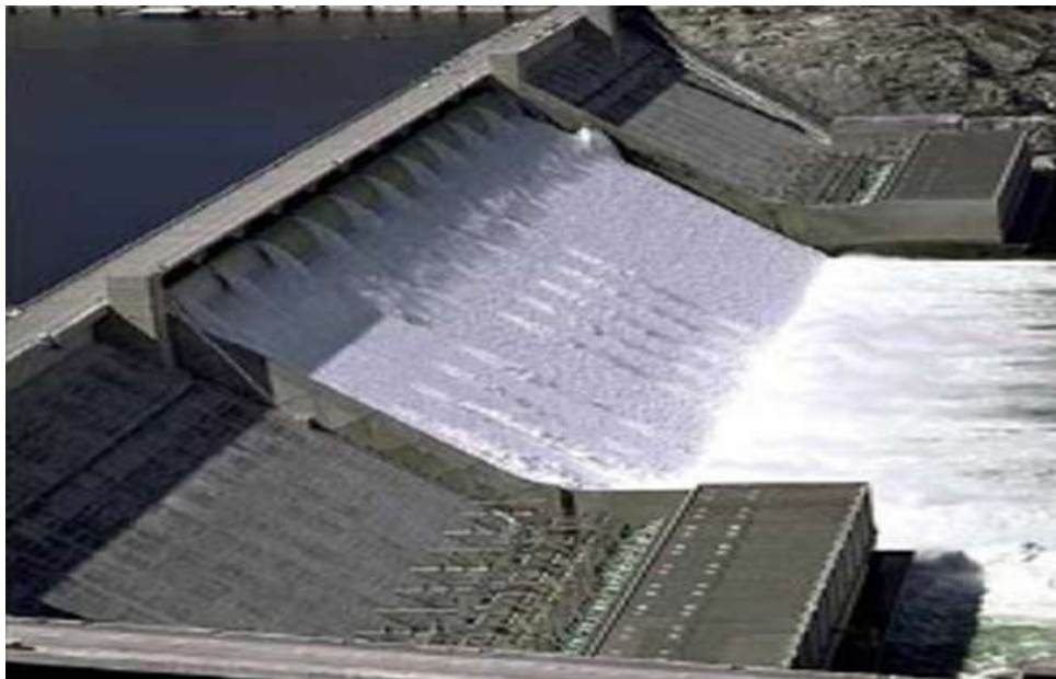
Concrete Gravity Dam with Overflow Section
