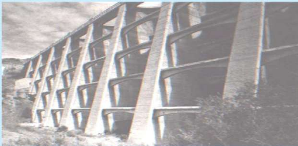
Buttress Dam (d/s side)
